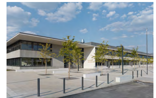
Elementary + High School, Stuttgart/Swen Carlin, Heidelberg
